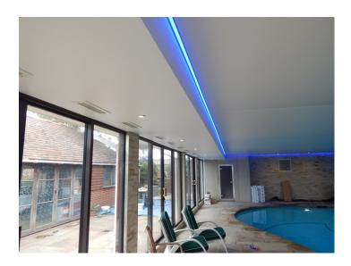
The finished ceiling with ducting wrapped, vents & downlights installed
