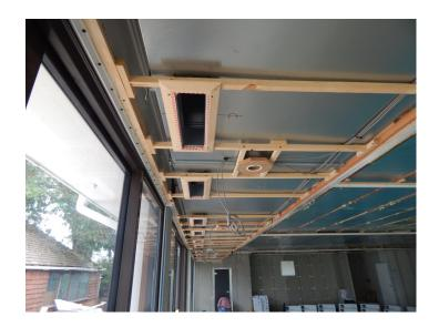
You will also notice the bosses installed so that apertures can be created in the ceiling membrane for the vents & down lights.
